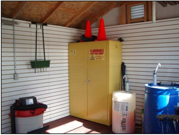
Fuel can storage cabinet
