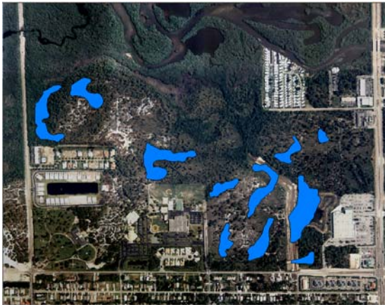
Final locations of water management lakes shown in perspective with original property.
