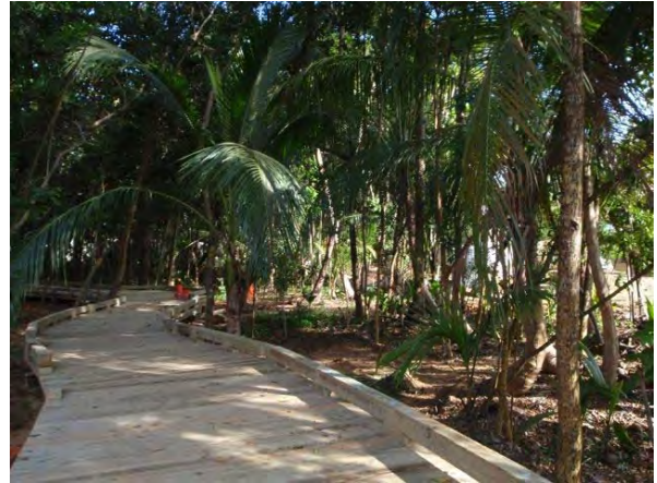
Elevated pathway under construction
