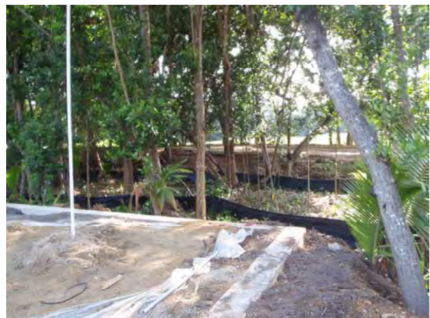
Rain garden by the St. Regis construction site
