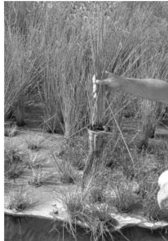
The floating mats consist of puzzle cut pieces held together by nylon connectors. Mats can be assembled in any size or shape. Emergent aquatic plants are inserted into pre-cut holes and quickly establish extensive roots.
