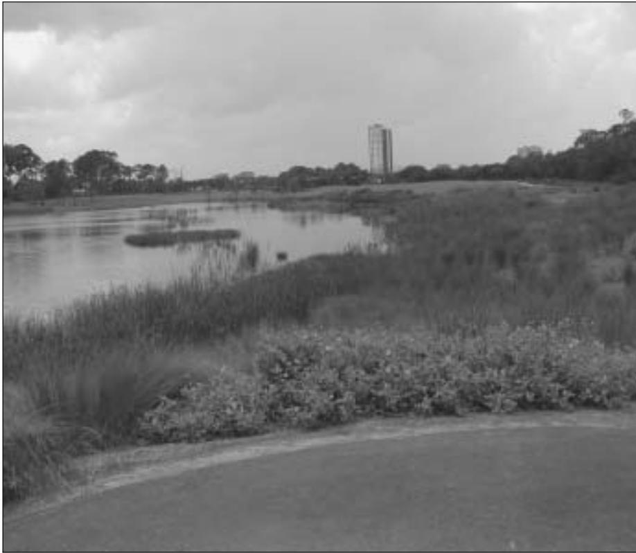
*When completed, the berm and gradually sloping shallow banks of the phytozones are vegetated with a variety of aquatic plants. The aquatic plants provide added water quality treatment by trapping solids and taking up dissolved nutrients.*
