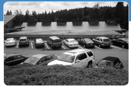
The visibility of the roof from the Glendale Country Club parking lot put aesthetics at the forefront of many decisions.
